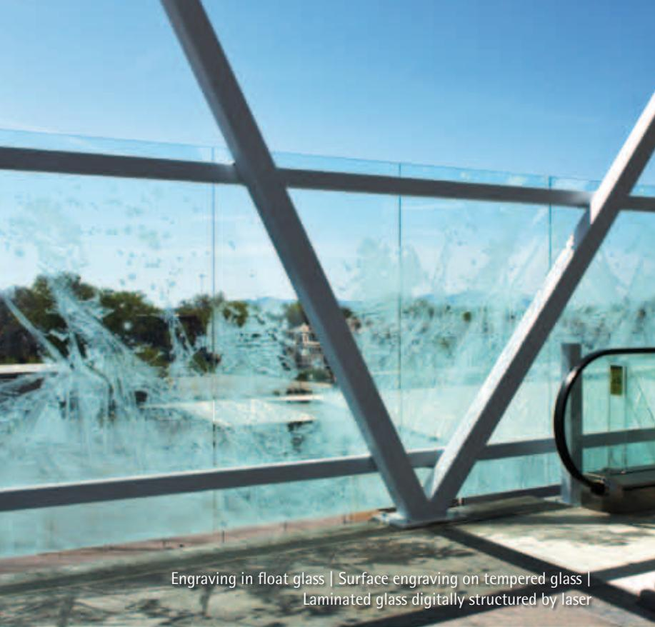
Engraving in float glass | Surface engraving on tempered glass |
